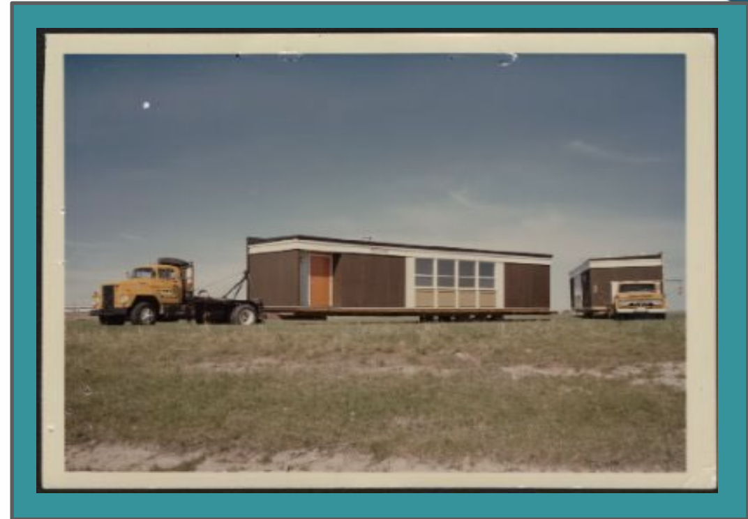
Prefabricated Day School being delivered to location, Forest, Ontario, ca. 1967, e011794878
